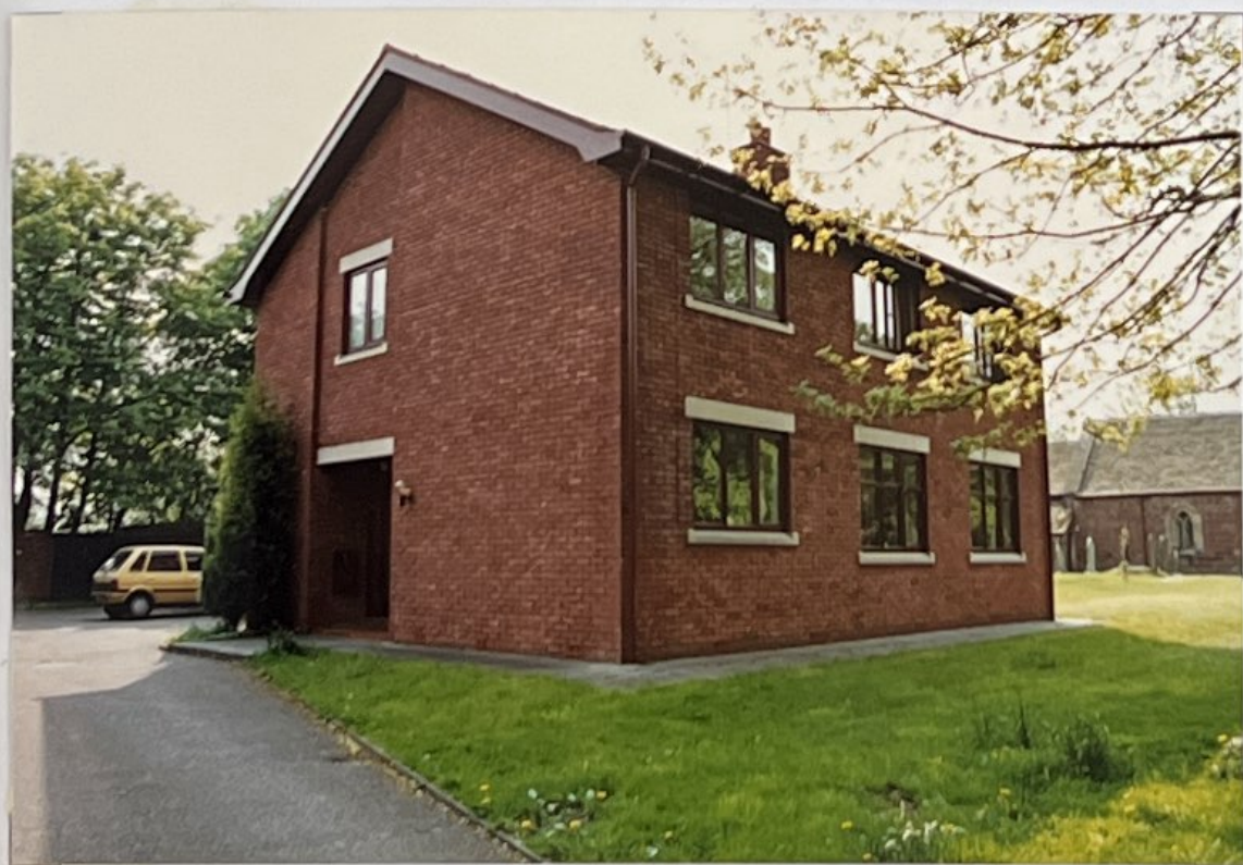
Front and side of the "new" vicarage.
